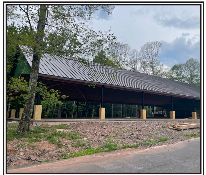
The Finished Pavilion Roof
