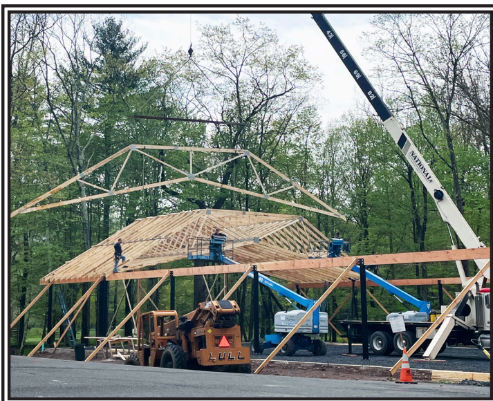
Installing the Trusses
