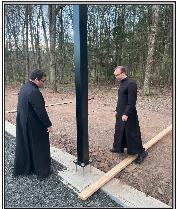
Inspecting the Pavilion Work
