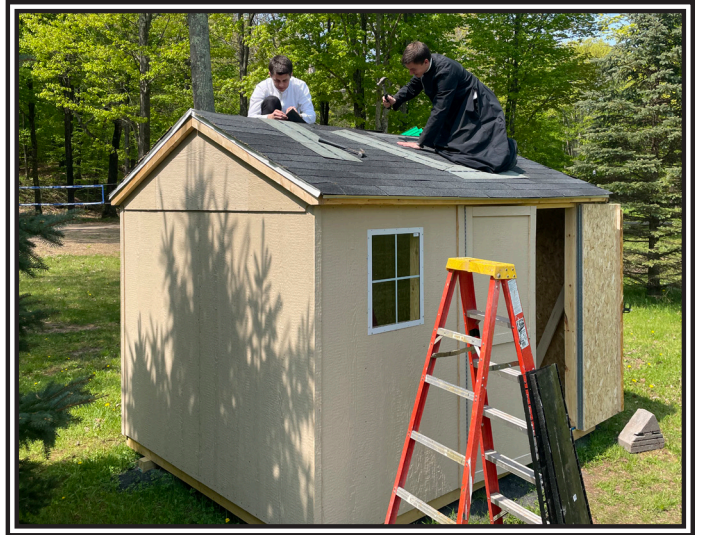
Roofing a New Storage Shed
